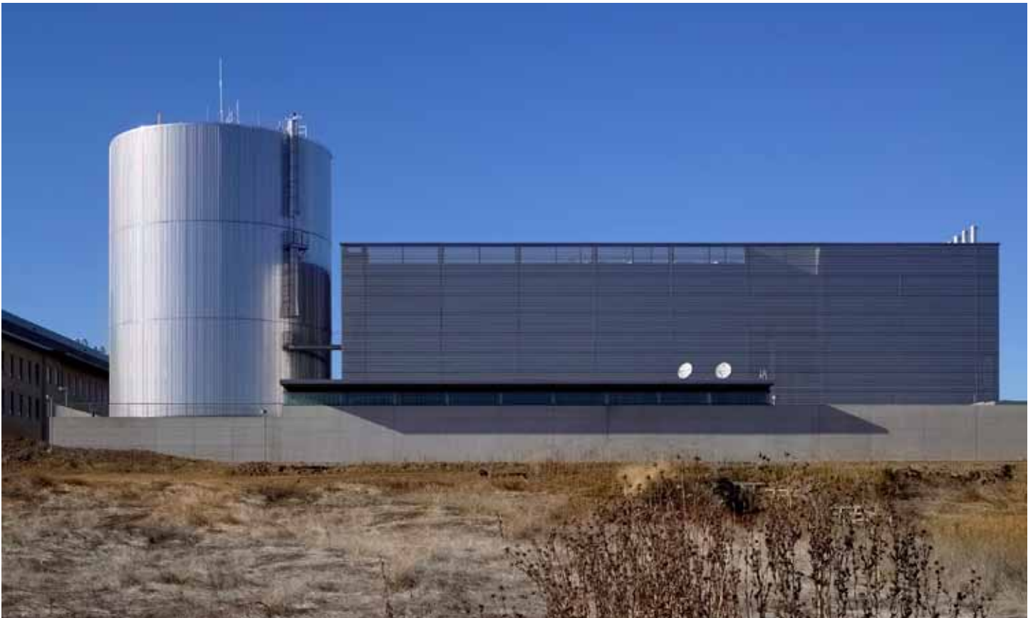
The Central Plant's northern elevation is perched over the edge of what will eventually be open space.
