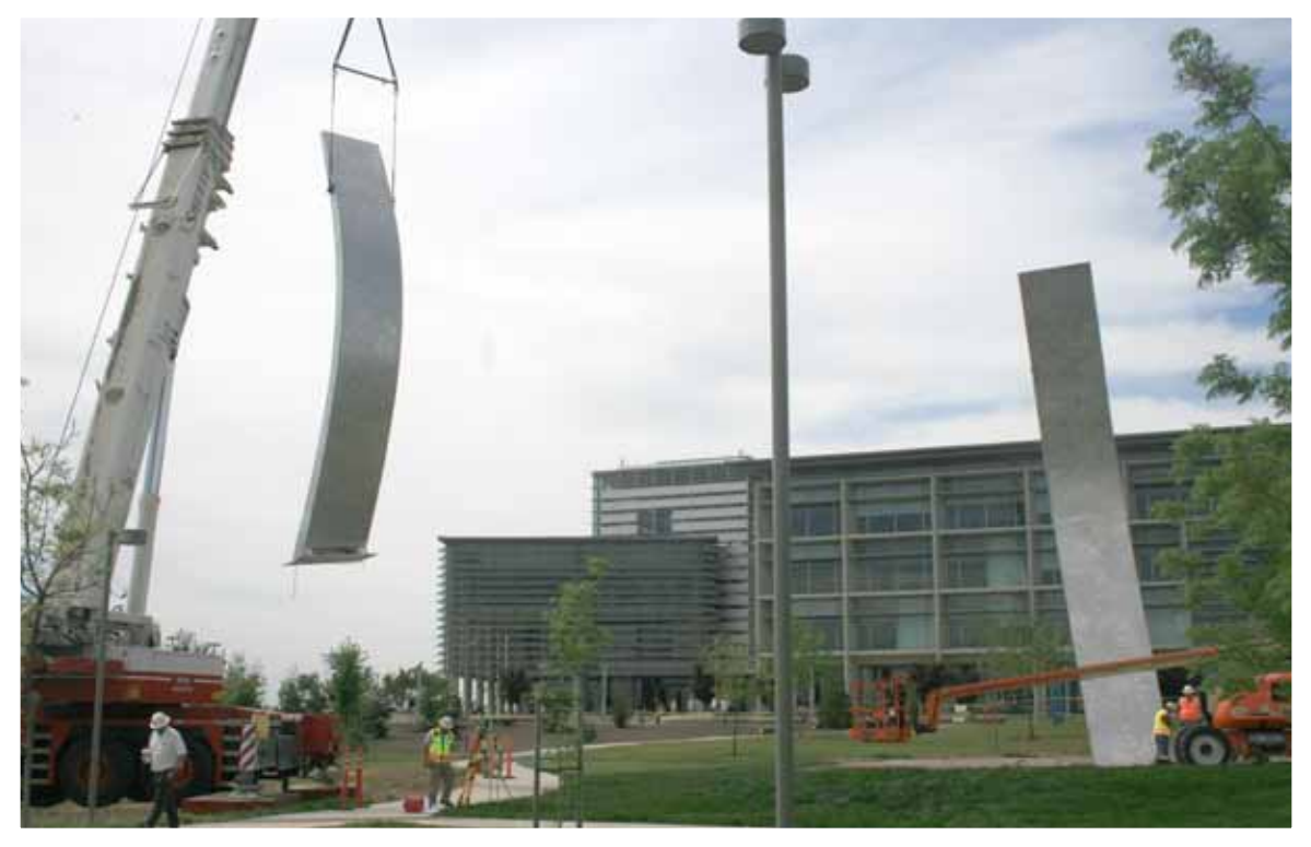
Installation of the 40-foot tall stainless steel components of the "Beginnings" sculpture, 2009.
