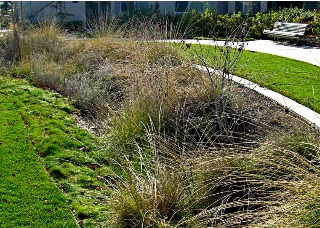
This example of a campus bioswale filters stormwater.
