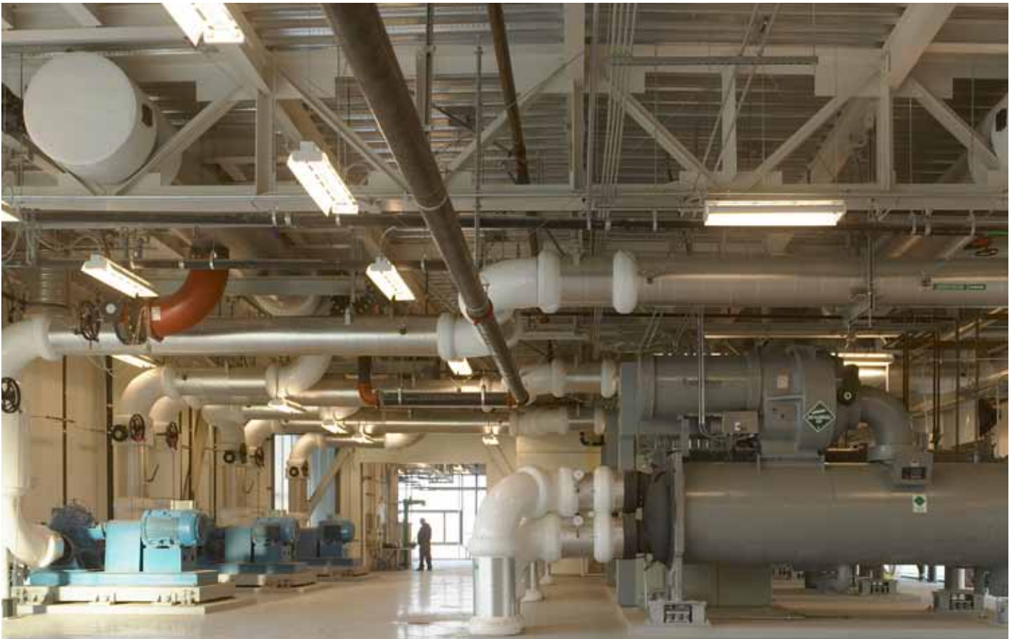
Inside the Central Plant, state of the art mechanical equipment forms the core of campus energy efficiency.
