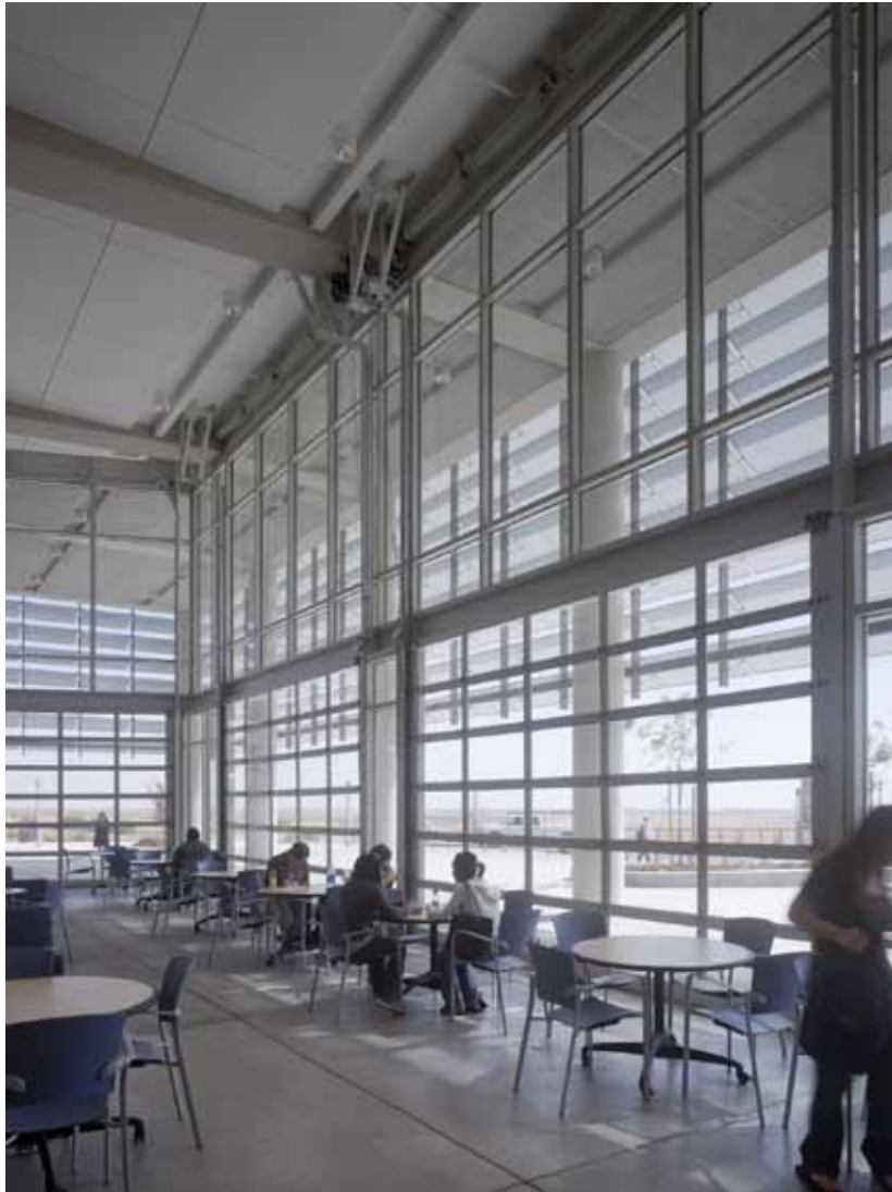
The ground floor of Kolligian Library is composed of full length glass walls that provide an engaging view of pedestrians on Scholars Lane. The walls can be rolled up for natural ventilation.
