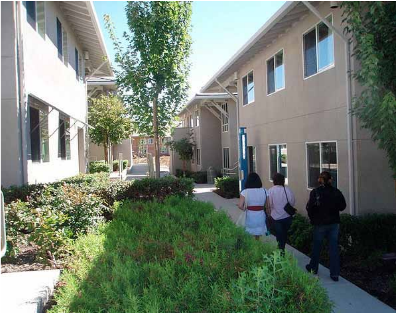
Strategic building siting and deep overhangs combine to cool building walls while shading windows and sidewalks. On hot days, the temperature differential between shaded and sunny areas can be up to 20 degrees fahrenheit.
