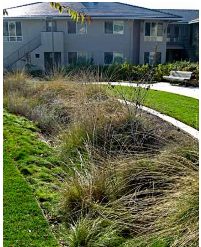
The Valley Terraces residences are composed of nine two-story buildings. Drought-tolerant bioswales have been integrated into the set of buildings in order to manage stormwater on-site
