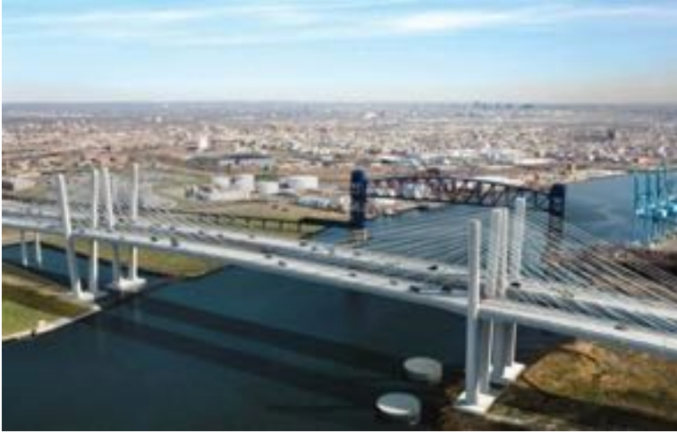
Goethels Bridge Replacement New York/New Jersey Opens 2018
