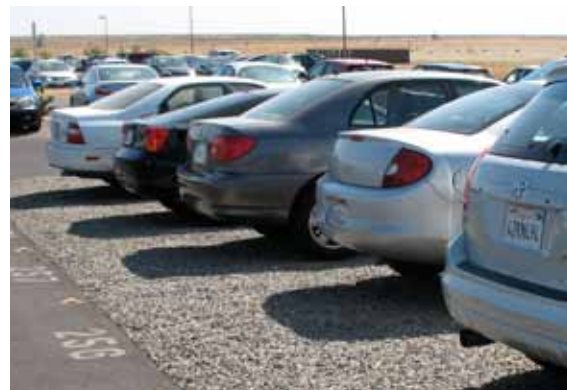
PERMEABLE SURFACES GROUNDWATER RECHARGE AND PARKING IN AREAS WHERE SOIL CONDITIONS PERMIT
