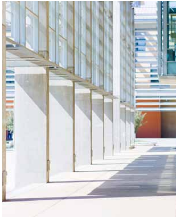
SCIENCE AND ENGINEERING 1 OVERHANG, SUN SHADES AND HEAVY MASS WALLS
